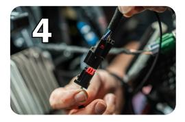
• Plug the male connector on the wire harness into the HVAC control panel and set it aside.
